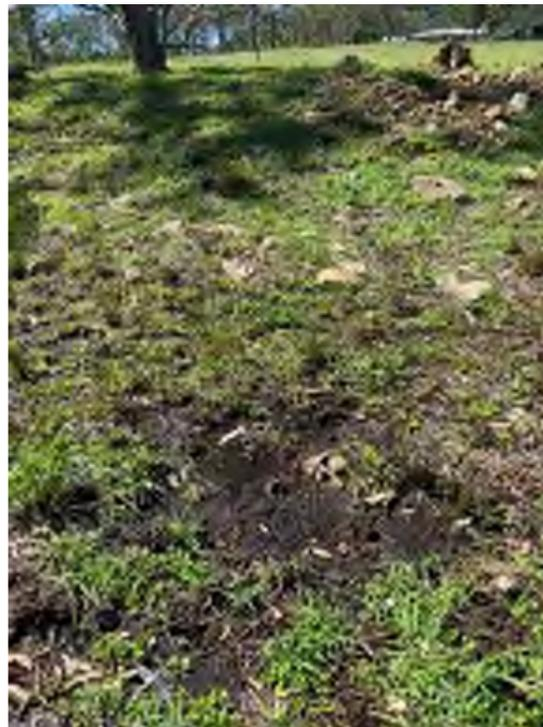
Photograph 5: View looking south east at the northern wall of Dam South showing dam seepage
